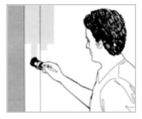
Apply adhesive to the wall and back of wall material with a brush corresponding to 150 mm on each side of the corner and allow drying within the actual adhesives open time. For this purpose a water based contact adhesive can be used.
