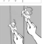
Welded seams must be allowed to cool to room temperature before they are trimmed. For best results, trim excess welding rod in two stages.
