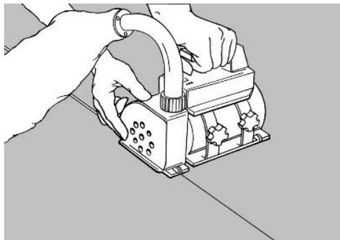
The sheets are hot welded. Do not weld until the adhesive has bonded completely, wait 24–48h. The joints are chamfered or grooved to about  $\frac{3}{4}$  of the thickness using a hand grooving tool or machine prior to welding.
